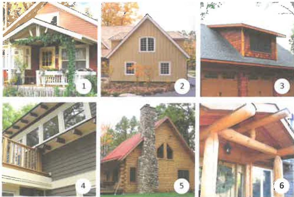
Figure: Examples of building design elements: Front porch (1); moderate sloping roof pitch (2); Dormer (3); Exposed rafters (4); Strong chimney element (5); and log pillars and beams (6).
