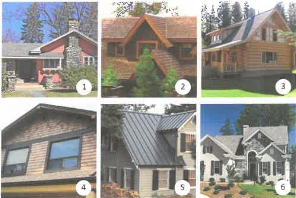
Figure: Examples of acceptable materials: Stone accents (1); natural wood trim (2); Log walls (3); Cedar shingles (4); Metal roof (5); and Stucco combined with other materials (6).
